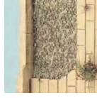
REN-E Render - existing Repaired & painted Location: Existing facade ornamentation
