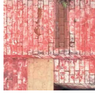
BE-E Brickwork - existing Existing paint stripped Location: Existing facades
