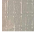
PM Pressed Metal (new) Location: Street awning soffit
