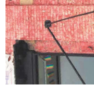
HS Steel members Paint Finish - protective coating Location: Awnings
